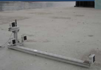
Measurement referential with LED targets in the south tower foundation
