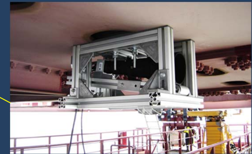
Camera (300 mm lens + converter) installed in the main span central section
