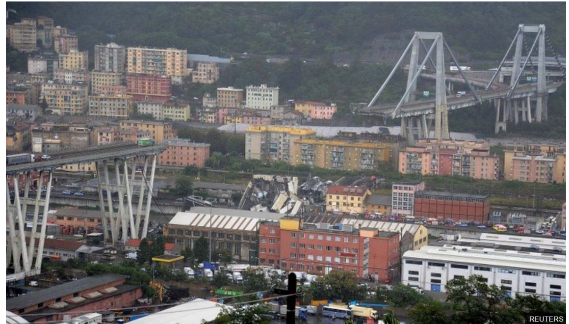
Morandi bridge Collapse in Genoa, Italy, Aug. 14, 2018 (photo: Reuters)
